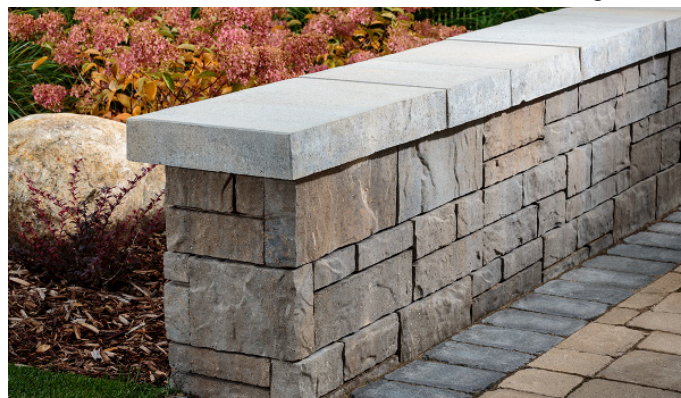
Example of Freestanding Landscape Walls
