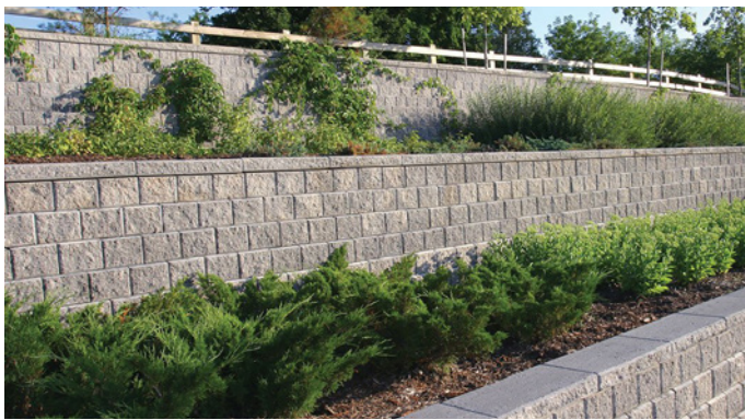
Example of Terraced Retaining Walls
