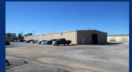
Paved parking/storage area
