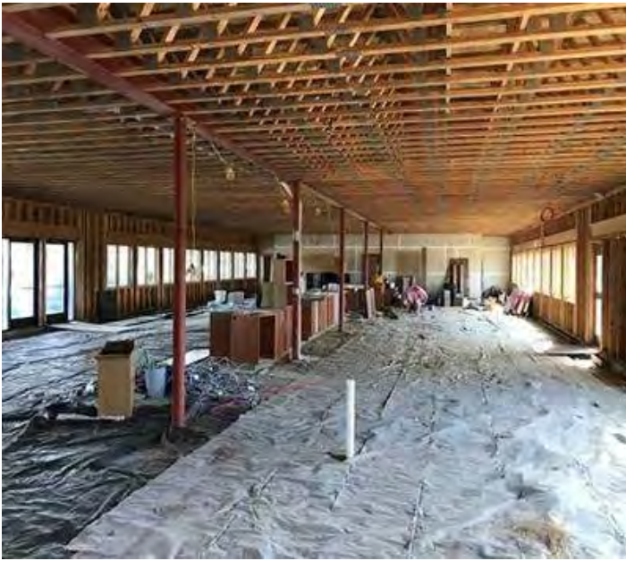
Wide Open and Ready to be Built Out
