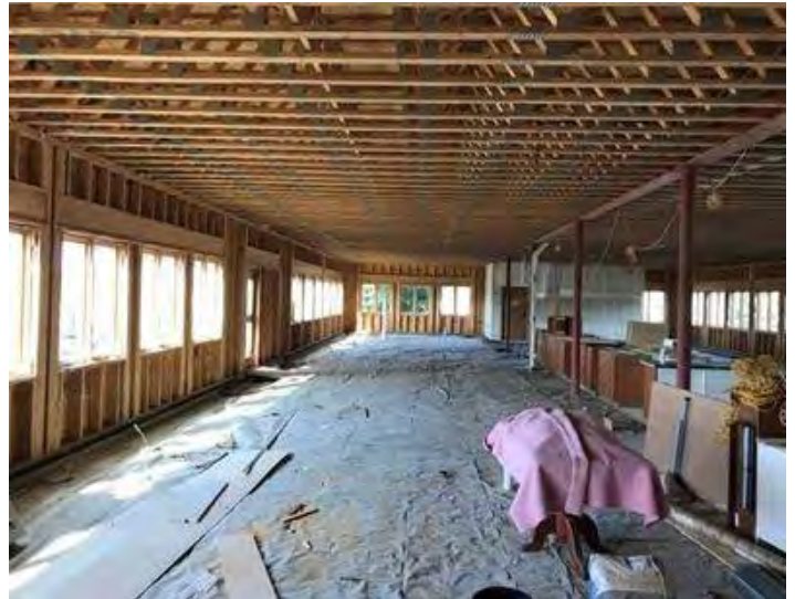
Windows Provide Plenty of Natural Light
