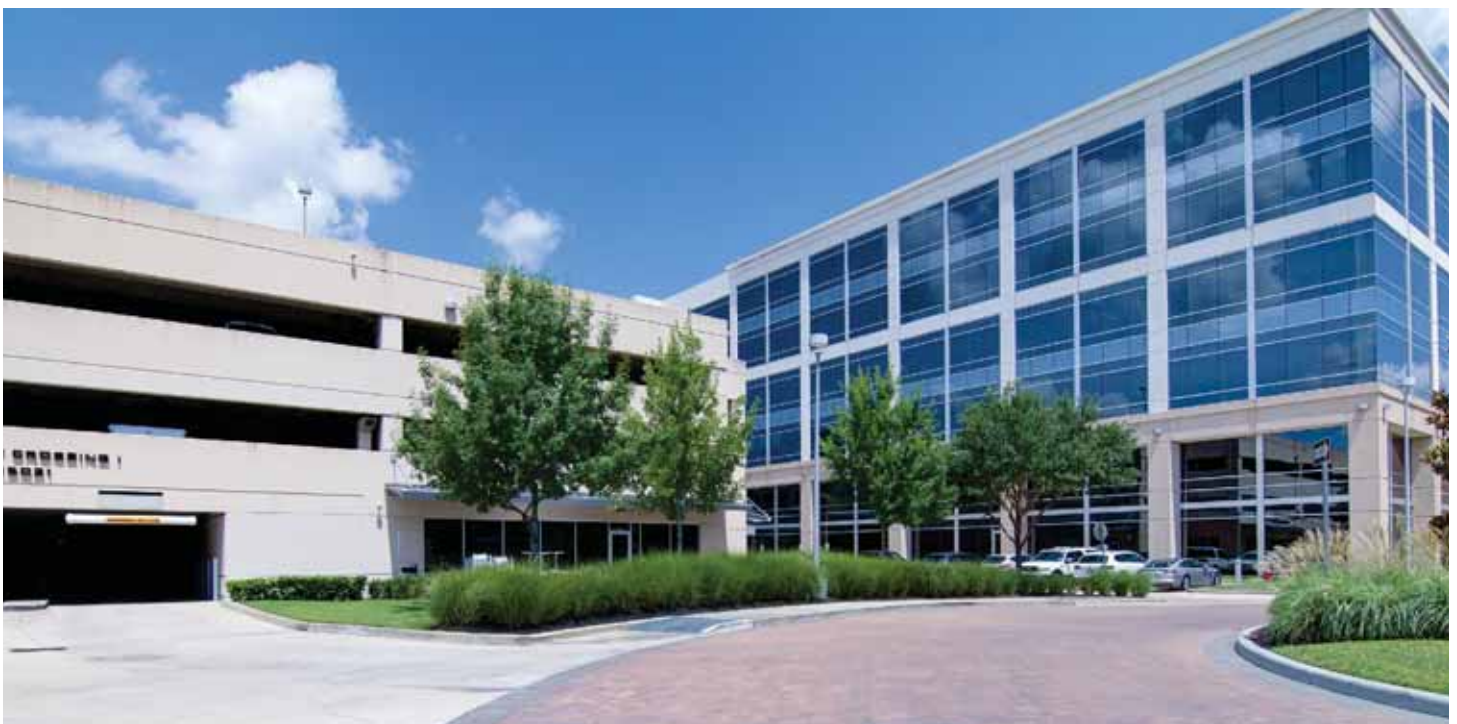
15021 KATY FREEWAY AND PARKING GARAGE
