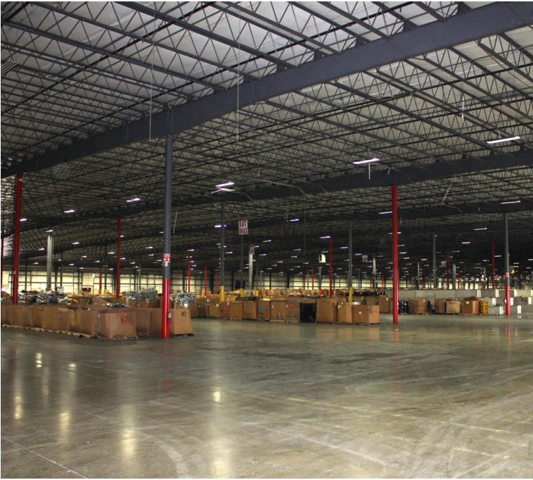
*Lighting recently upgraded to T-5 with motion sensors
