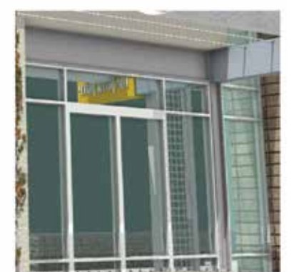
storefront system Clear anodized aluminum storefront systems with green tinted glass and spandrel glass
