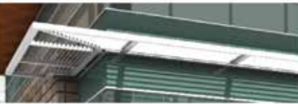
shade trellis Steel structure and angled louvers create filtered shade
