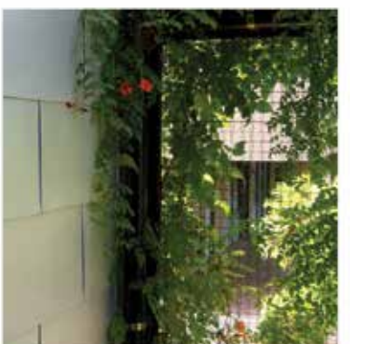
greenscreen Steel structure and "greenscreen" mesh in fill creates living screen walls of vines
