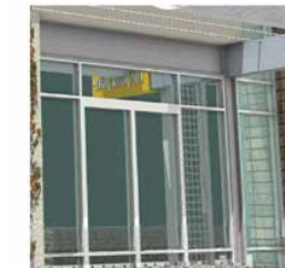
storefront system Steel structure and aluminum storefront systems with green tinted glass and spandrel glass
