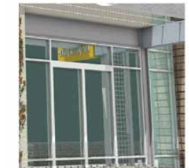
storefront system Clear modulated aluminum storefront systems with green tinted glass and spandrel glass
