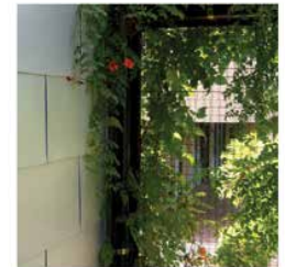
greenscreen Steel structure and "greenscreen" mesh in fill creates living screen walls of vines
