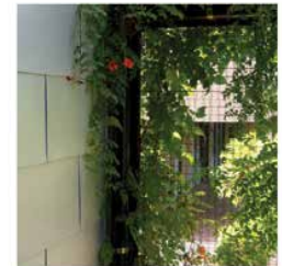
greenscreen Steel structure and "greenization" mesh in fill creates living screen walls of vines
