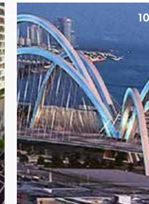
10 SIGNATURE BRIDGE Will carry a key segment of I-395 over NE 2nd Avenue and Biscayne Boulevard and redefine the Miami skyline with its six sweeping arches.
