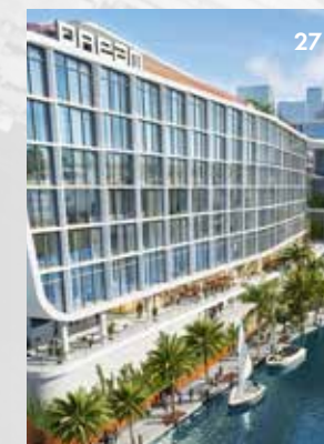
27 RIVERSIDE WHARF Riverside Wharf is a major mixed use project slated for two towers of development, 90,000 SF of entertainment space and 165 Hotel units.
