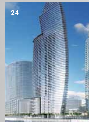
24 ASTON MARTIN RESIDENCES Aston Martin Residences, currently under construction, is a 66-story luxury condo tower with 391 units. The building will feature a full service marina that can accommodate superyachts.
