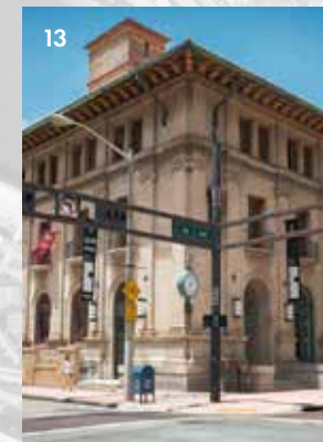
13 POST OFFICE FOODHALL Stambul USA will turn building into food and beverage complex with a Mexican restaurant, Biscayne Bay Brewing, juice bar and other offerings.
